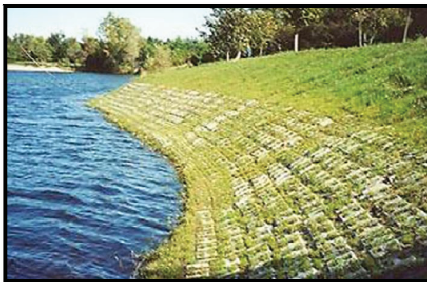
Picture 7. Installed of Fabric Formed Concrete with Grass Growing Through It
