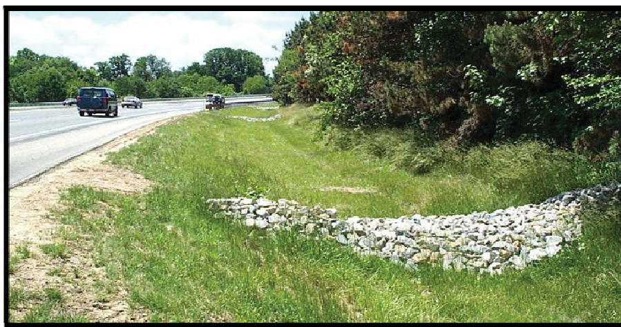
Picture 4. Example Picture of Rock Check Dams
