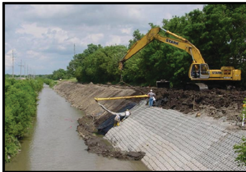
Picture 5. Installation of Fabric Formed Concrete for Erosion Protection
